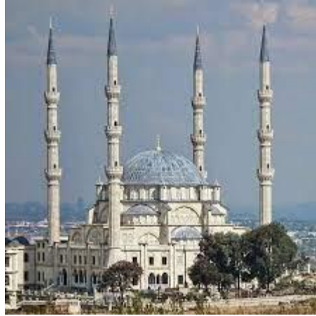
Figure 2.24: Nizamiye Mosque in Midrand, Johannesburg
